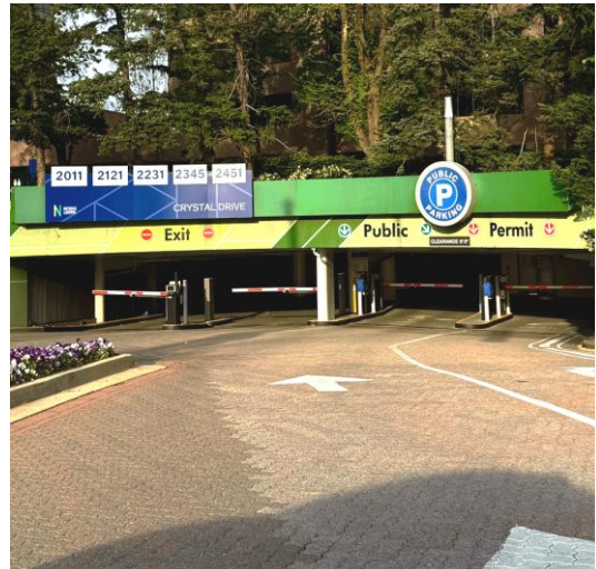
2345 Parking garage entrance
